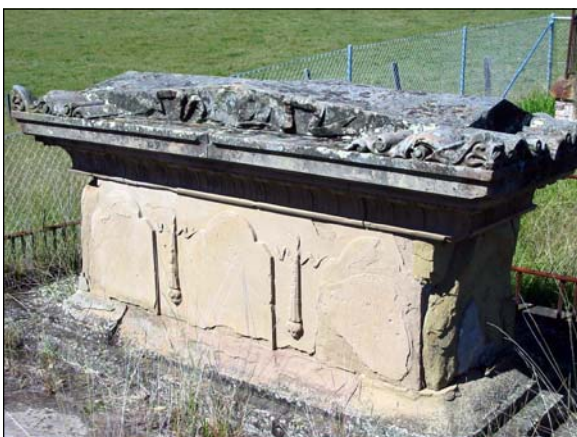
Weathered remains of the Clift Vault.
